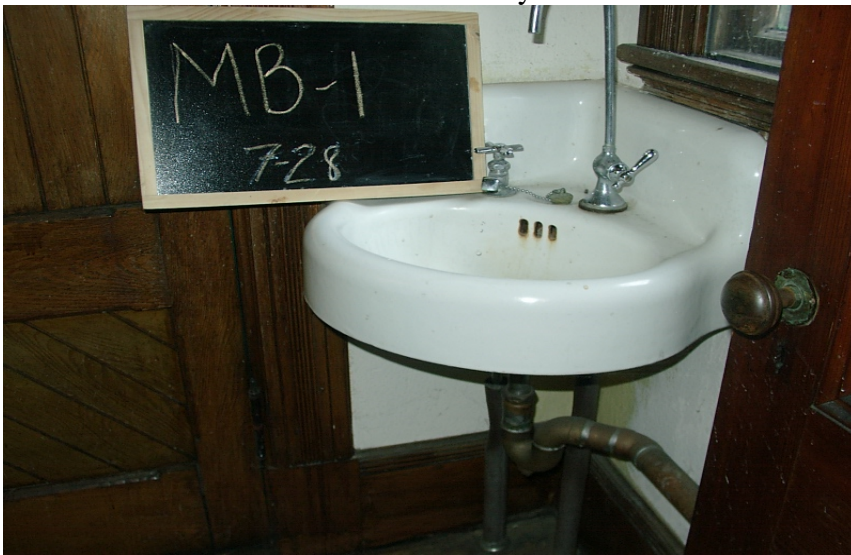
Memorial Bldg 1 st floor Faucet in hallway ( not functioning properly; leaks)
