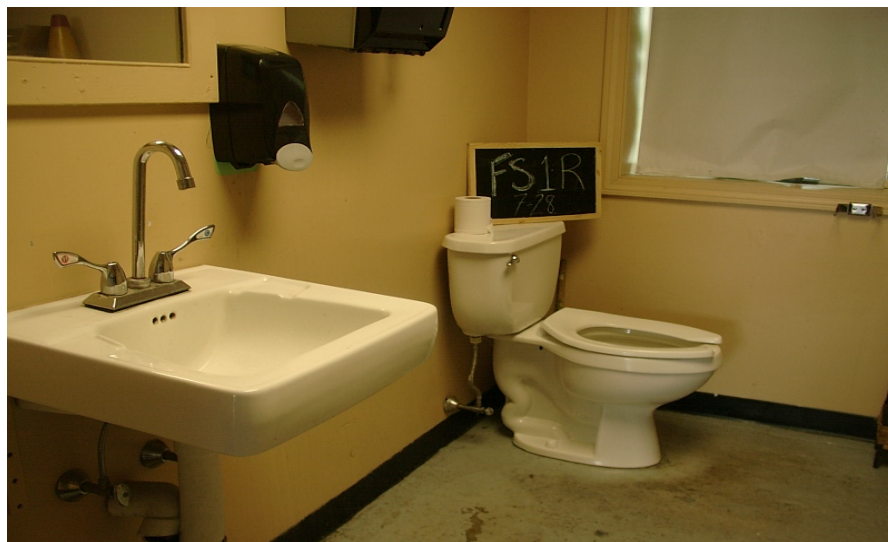
Fire station 1 st floor Unisex bathroom on the right hand side with 1 toilet and 1 sink (Not handicap accessible; no bar on the side of the bathroom, no ramp on the doorway and the faucet is not working properly)
