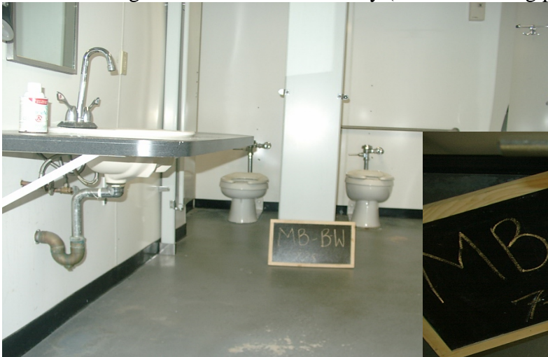
Memorial Bldg Basement (toilet 1.6 gallon tank – newer model)
